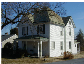
Little High Street Area 320 11th Street Assessment: $320,000 Built: pre-1920
